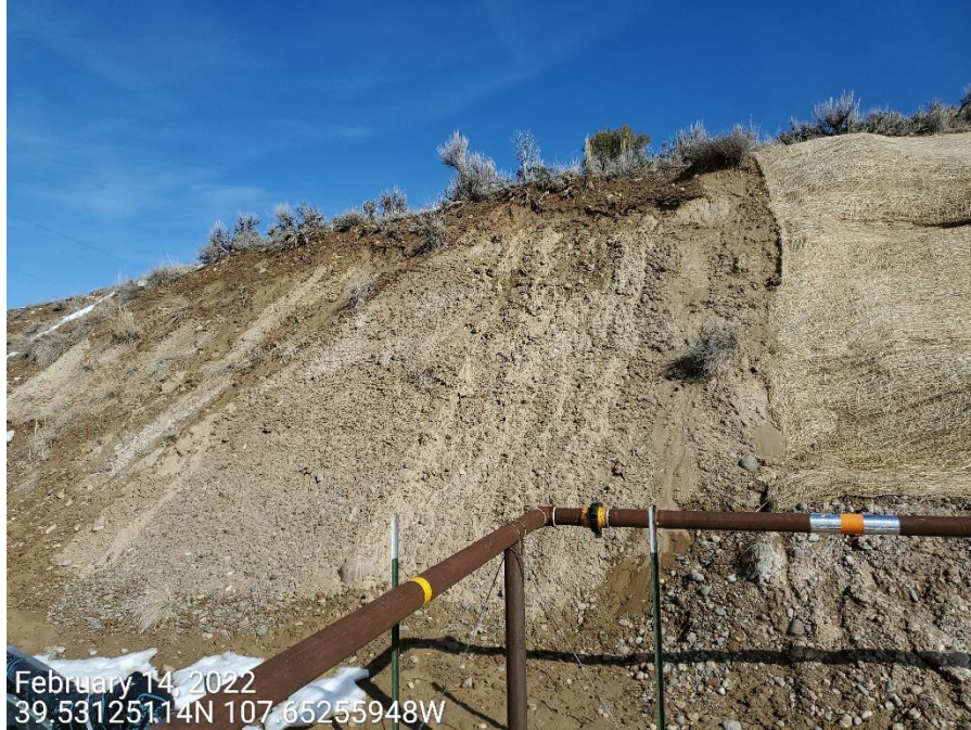
Photo 2: Photos taken from the cut slopes. Photos provide examples showing control measures to protect/stabilize the cut slopes of the Location remain missing or insufficient; erosion degradation evident.
