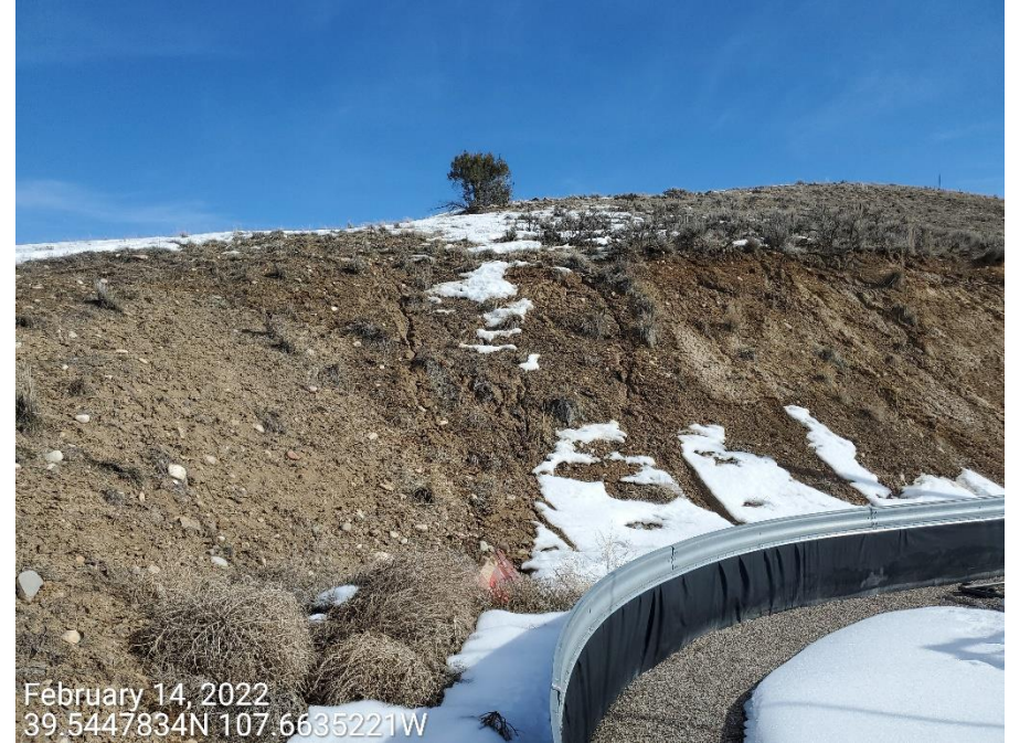
Photo 2: Photos taken from the cut slopes. Photos provide examples showing control measures to protect/stabilize the cut slopes of the Location remain missing or insufficient; erosion degradation evident.
