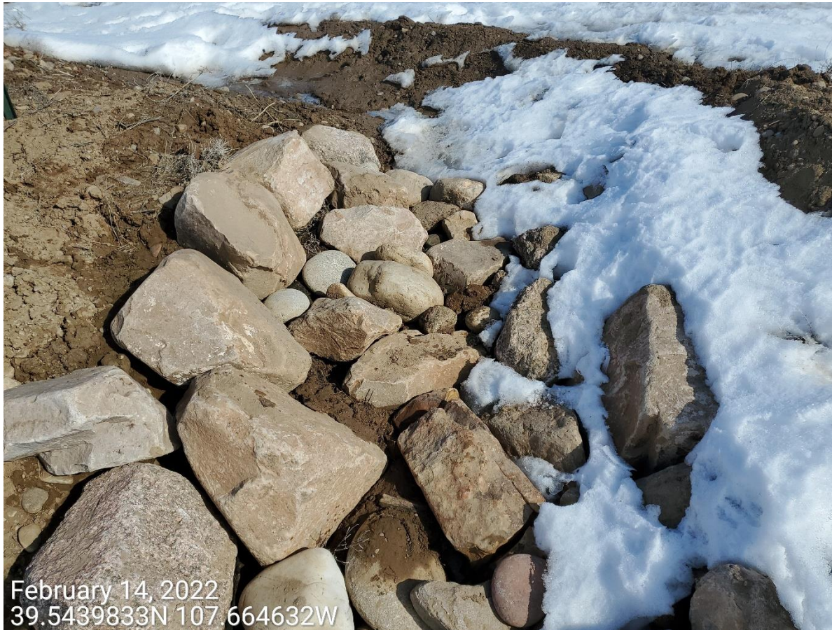
Photo 4: Photo taken from the outlet on the west end of the Location; outlet has been re-installed with rip-rap and geotextile armoring.
