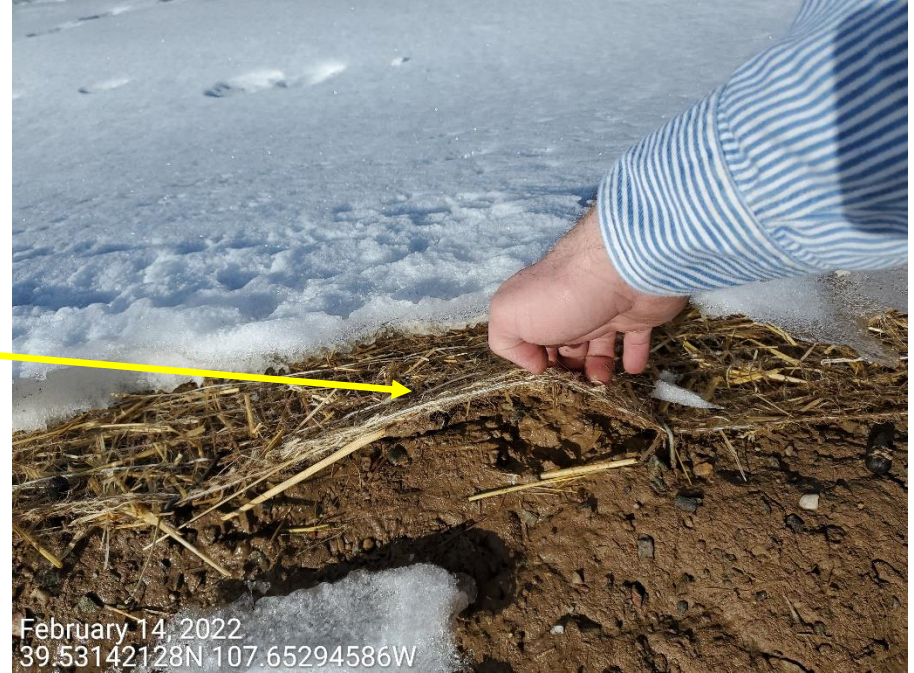
Photo 3: Photos taken from the slopes on the north end of the Location. Photo example showing that the blankets installed on the Location have not been installed in accordance with good engineering practices; blankets have not been properly trenched/anchored and backfilled.
