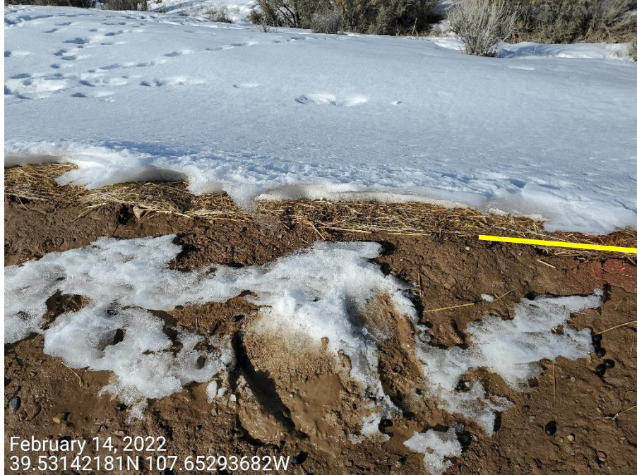
Photo 3: Photos taken from the slopes on the north end of the Location. Photo example showing that the blankets installed on the Location have not been installed in accordance with good engineering practices; blankets have not been properly trenched/anchored and backfilled.
