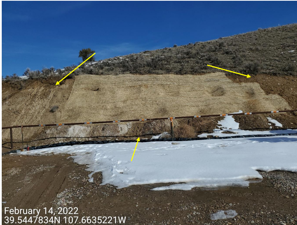
Photo 1: Photo taken from the east end of the Location, facing east. Photo shows Operator has implemented erosion control blankets on only a single section of the upper cut slopes of the Location. Control measures to protect and stabilize the remaining cut slopes left and right of the blanket seen in the photo, as well as slopes below the blanket.
