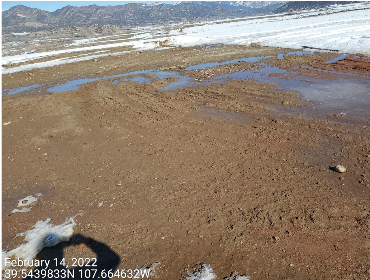
Photo 3: Photo taken from the western production area, facing northeast. Areas of the production pad not covered with snow do not appear to be stabilized, and are at risk of vehicle tracking and sediment transport.
