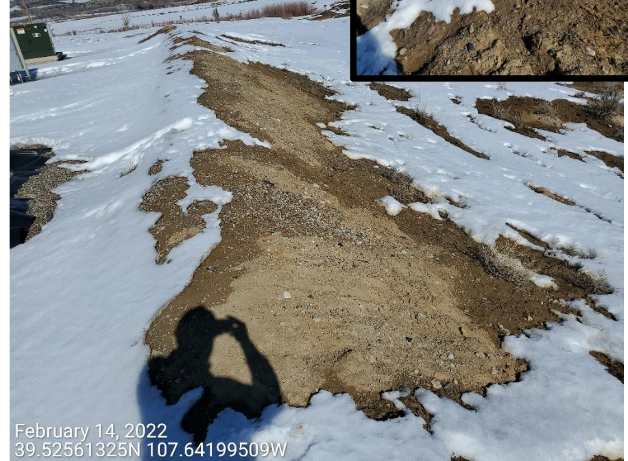
Photo 2: Photos taken from exposed areas of the cutslopes (photo left) and the eastern slopes of the Location (photo right). Unable to find evidence that control measures to protect and stabilize the slopes of the Location were installed or maintained. Photo insert top-right shows areas where rill erosion is evident on the eastern slopes.
