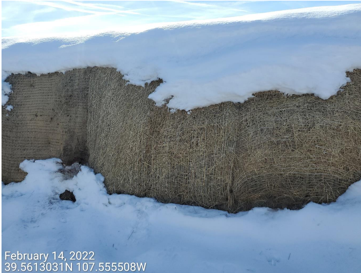
Photo 1: Photo taken from the cut slopes behind the separator equipment; erosion blankets have been maintained.
