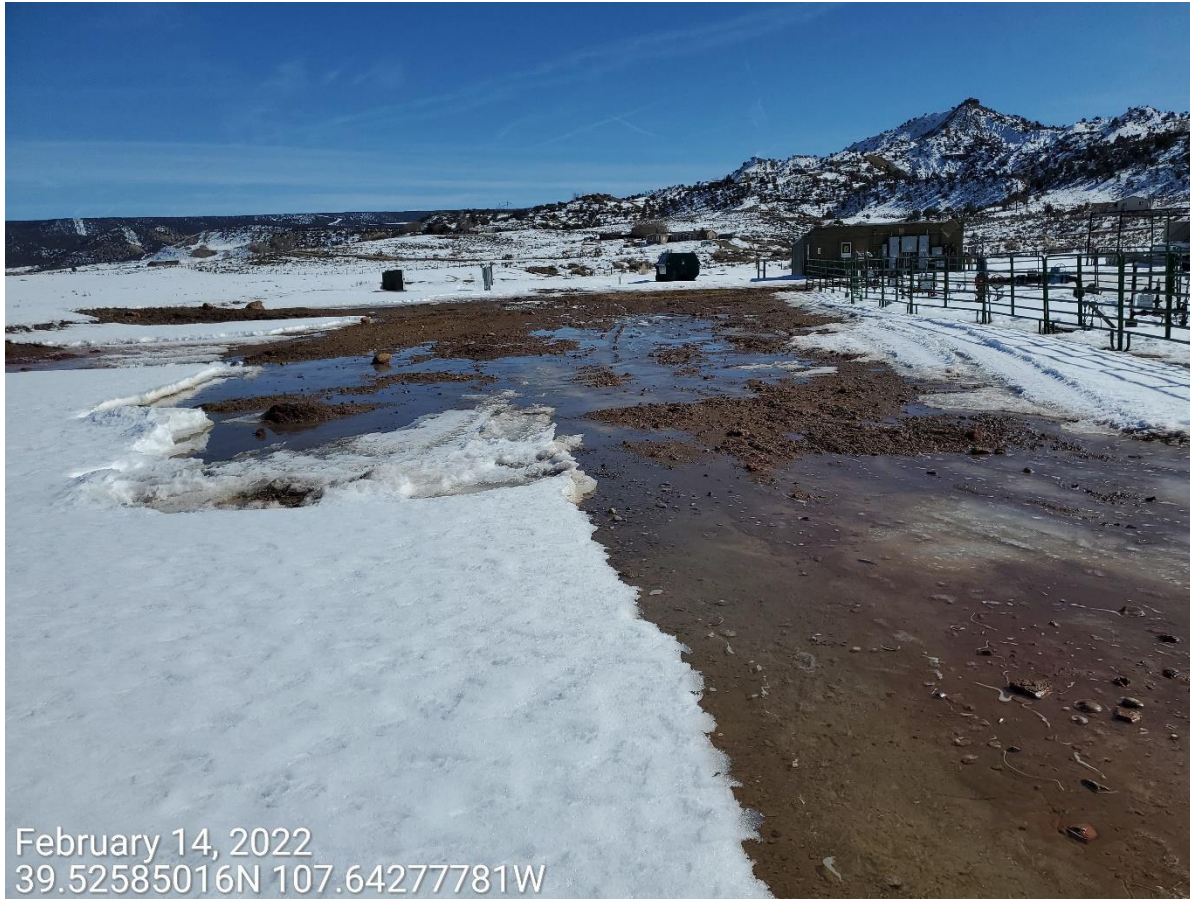
Photo 5: Photo taken from the northern end of the production area, facing south east. Areas of the production pad not covered with snow do not appear to be stabilized, and are at risk of vehicle tracking and sediment transport.
