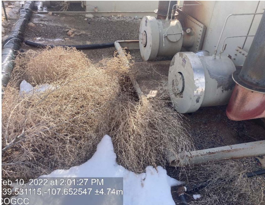
Debris (tumbleweeds) next to burners on separators that are running.
