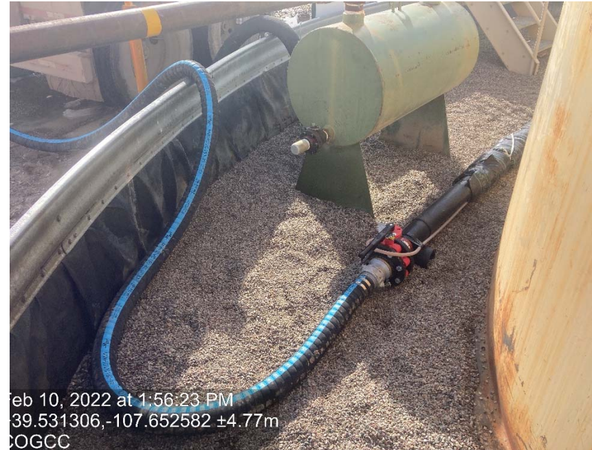
Truck loading fluid from valves at back of tanks, not the valves in the buckets.
