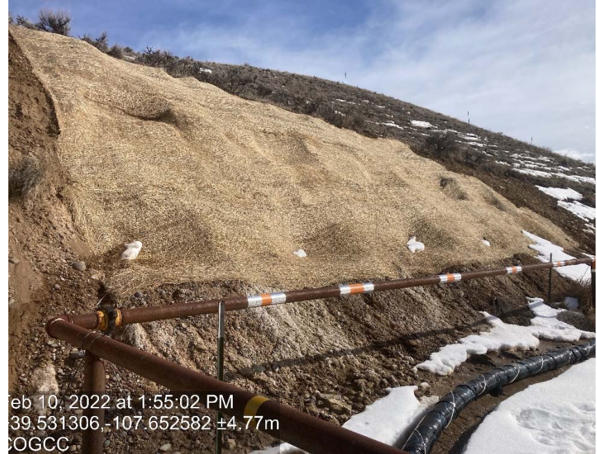
Some of cut slope has a blanket
