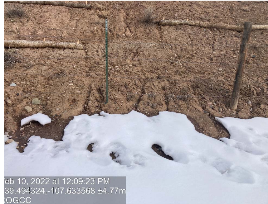
Cut slope lack of stabilization/erosion/riling
