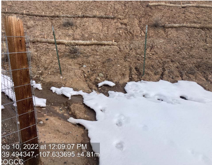
Cut slope lack of stabilization/erosion/riling
