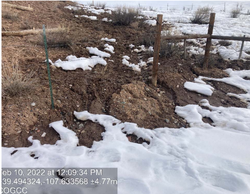
Cut slope lack of stabilization/erosion/riling
