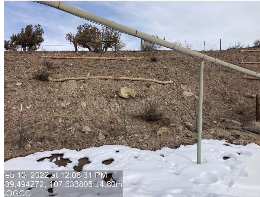
Cut slope lack of stabilization/erosion/riling
