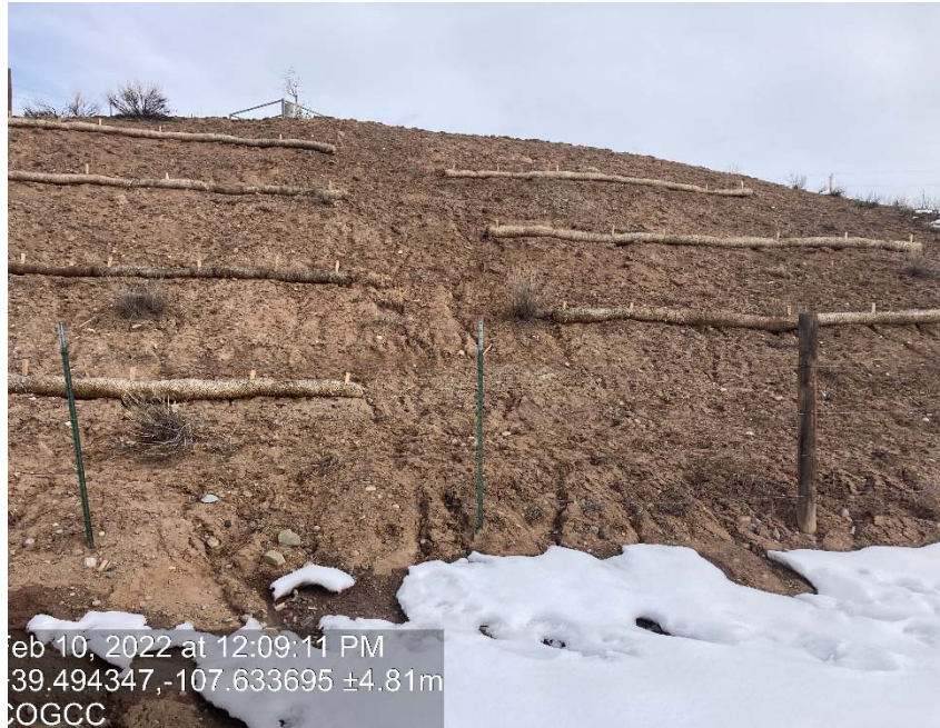
Cut slope lack of stabilization/erosion/riling
