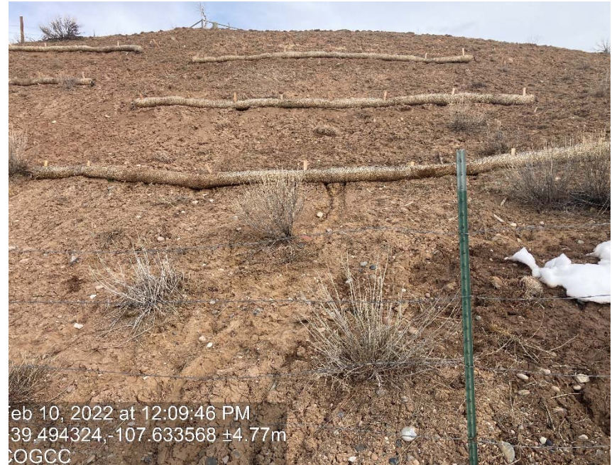
Cut slope lack of stabilization/erosion/riling
