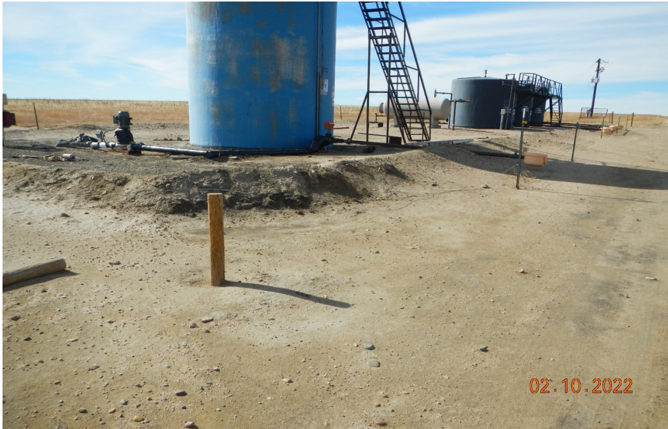
Photo 1. Facing toward the associated tank battery located 650 ft. north of the wellsite. The fence around the tank battery is not maintained and the earthen berms are not adequately sized to contain a spill.
