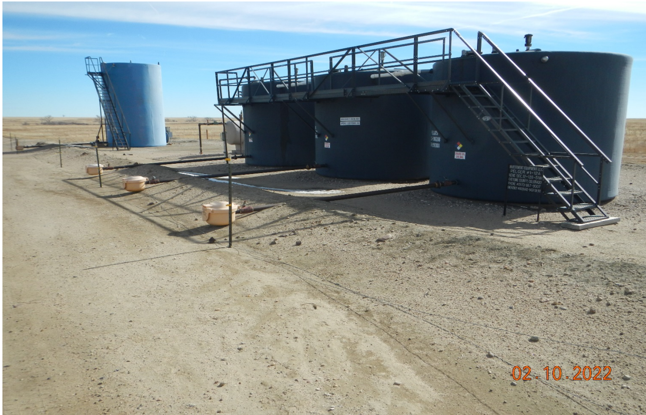
Photo 2. Facing toward the associated tank battery located 650 ft. north of the wellsite. The fence around the tank battery is not maintained and the earthen berms are not adequately sized to contain a spill.
