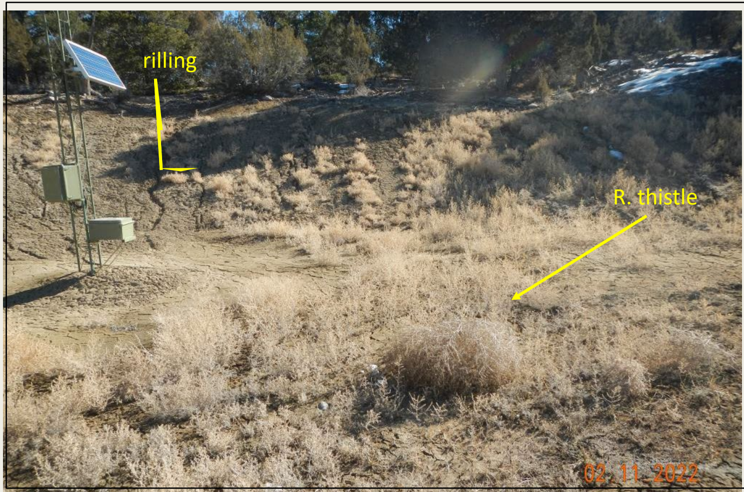
Photo 3. View of the eastern cut-slope. Rilling observed in several areas, up to approx. 10 inches deep. Little desirable vegetation observed. Bare soils are eroding. Russian thistle debris present.
