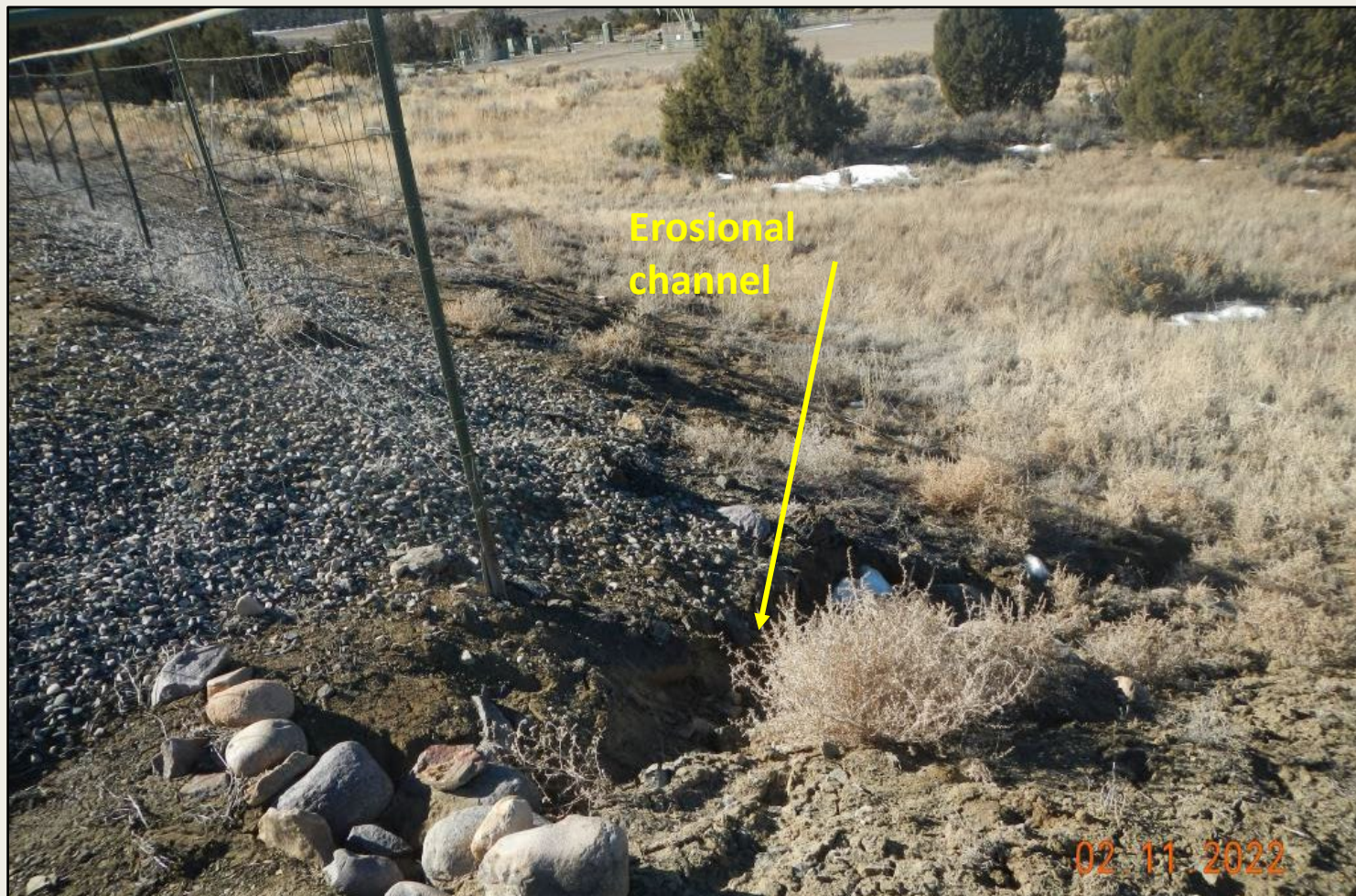
Photo 5. View of erosional channeling approx 2ft wide and deep in the northwestern project area. Cobble BMP is not adequate and no longer functioning as it is full of sediment.
