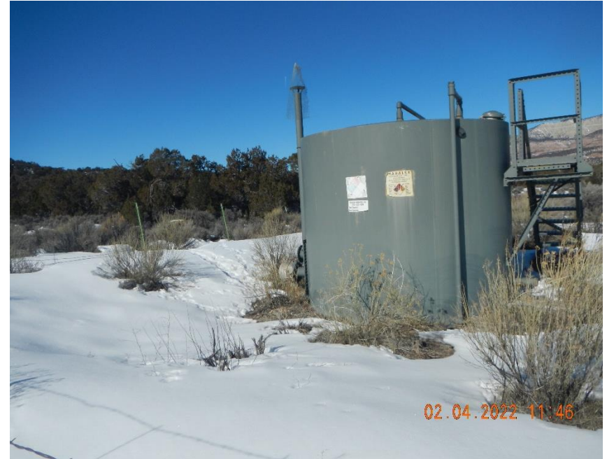
Tank capacity, contents and NFPA label weathered and not legible.
