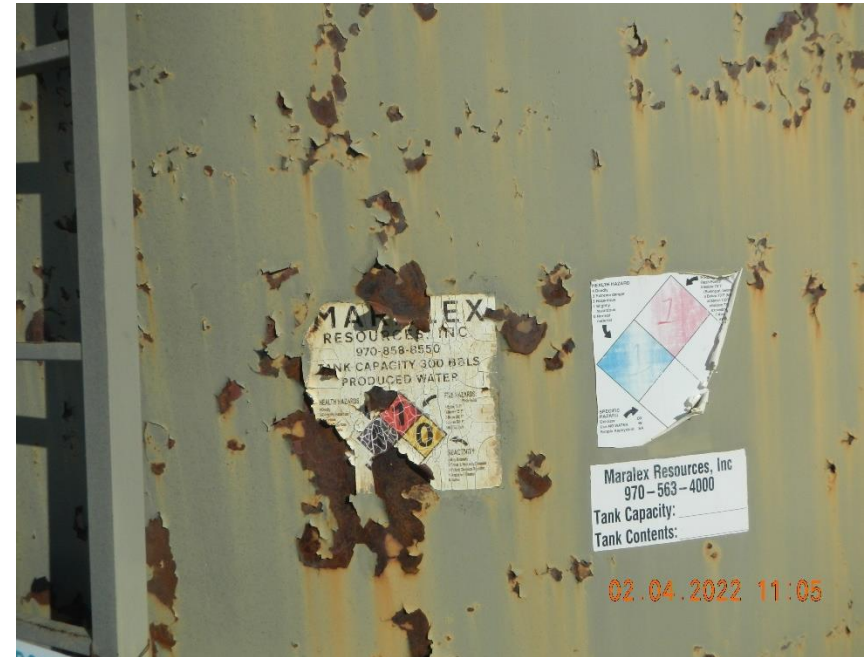
Tank label and placards are weathered and not legible.
