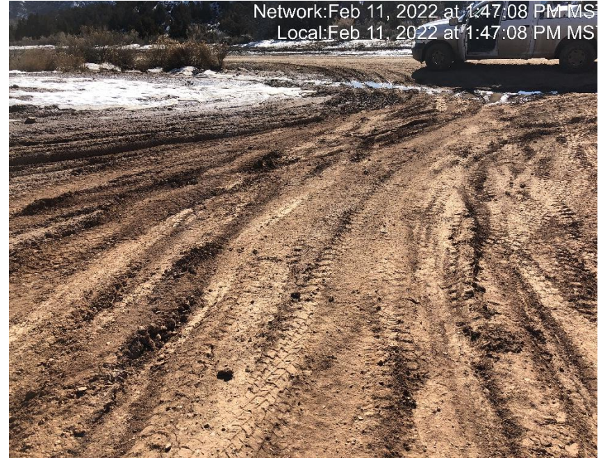
Photo #5947 Insufficient tracking BMP located at entrance to location.
