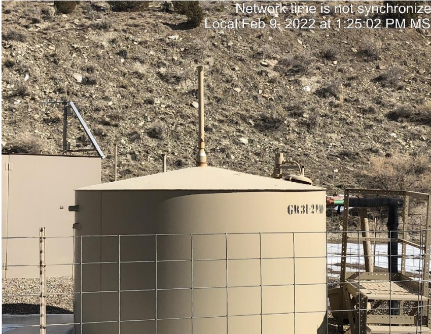
Photo #5920 Vent pipe on tank open ended.
