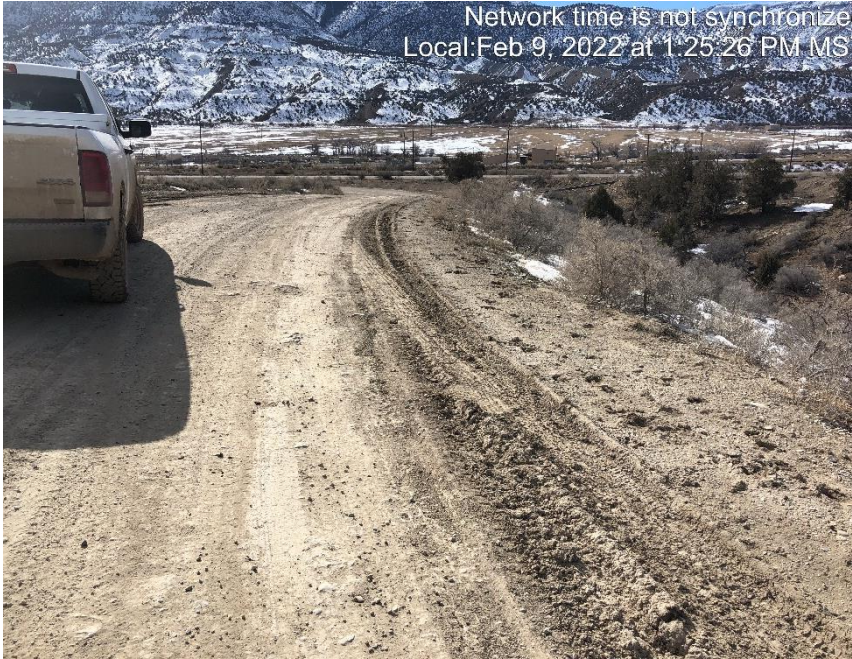
Photo #5923 Insufficient tracking BMP located at entrance to location.
