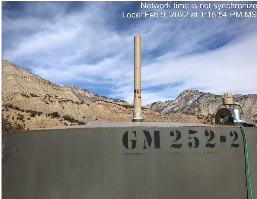
Photo #5910 Vent pipe on tank open ended.
