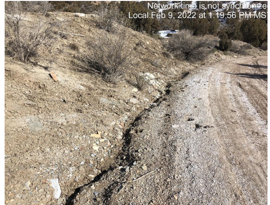
Photo #5914 Insufficient velocity checks.
