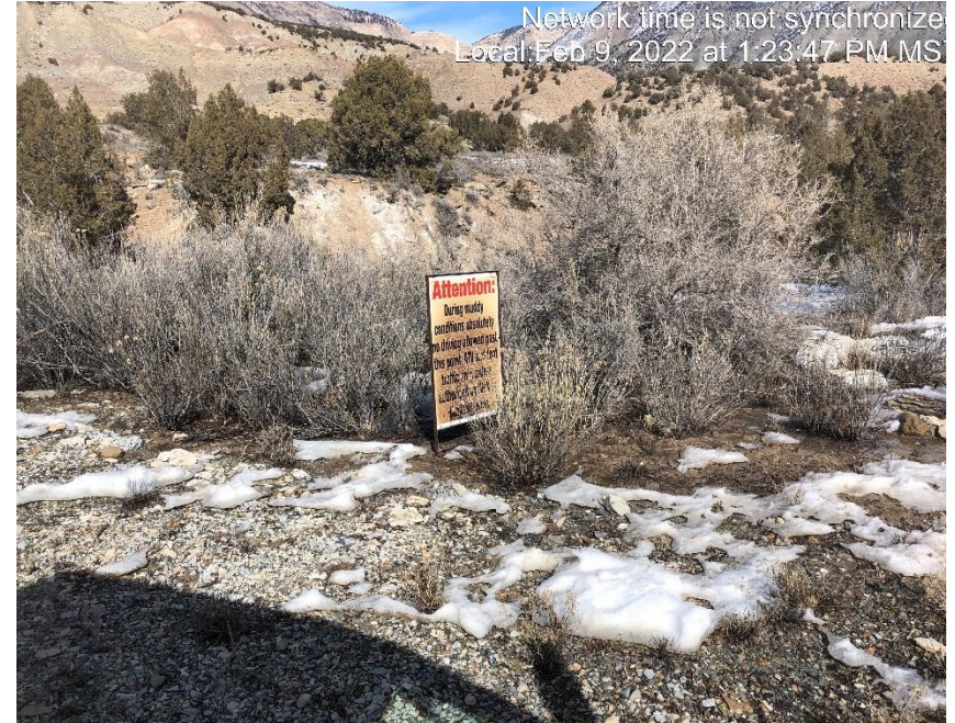
Photo #5917 Insufficient tracking BMP located at entrance to location.
