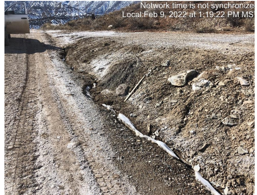
Photo #5911 Rill erosion occurring in ditch.
