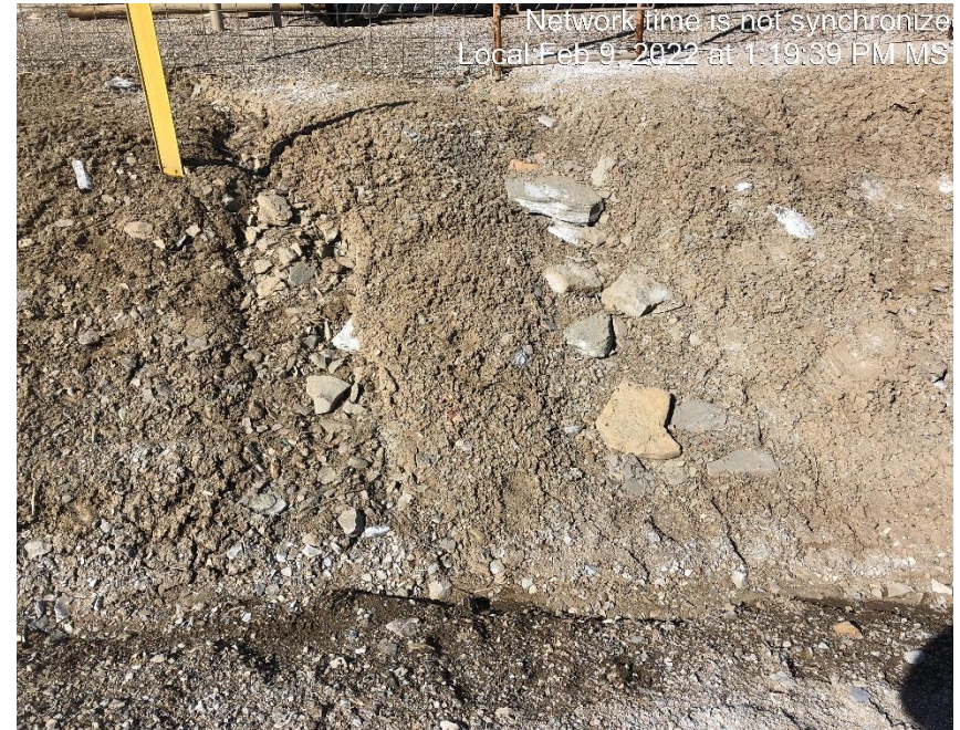
Photo #5913 Rill erosion occurring on berm.
