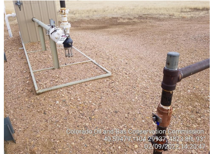
Photo 10 – Valve to Gas Sales – LOTO, Gas to ECD Open
