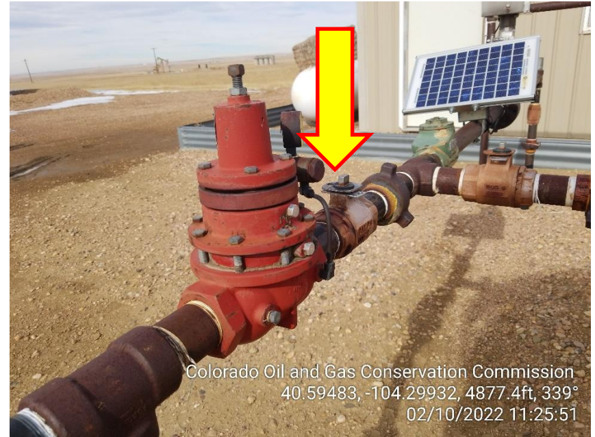
Photo 6 – Valve Open going to ECD
