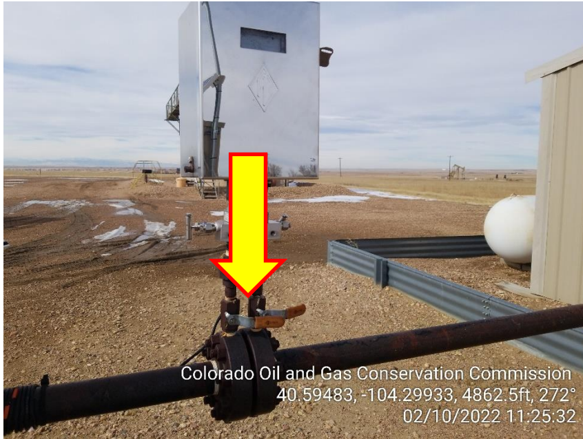
Photo 5 – Valves Closed at Gas Meter going to ECD
