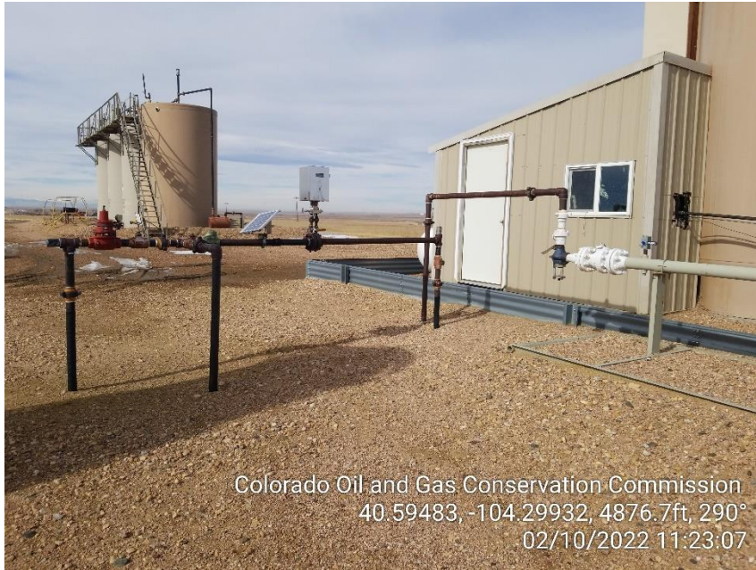
Photo 1 – Gas Lines – Going to Sales and ECD
