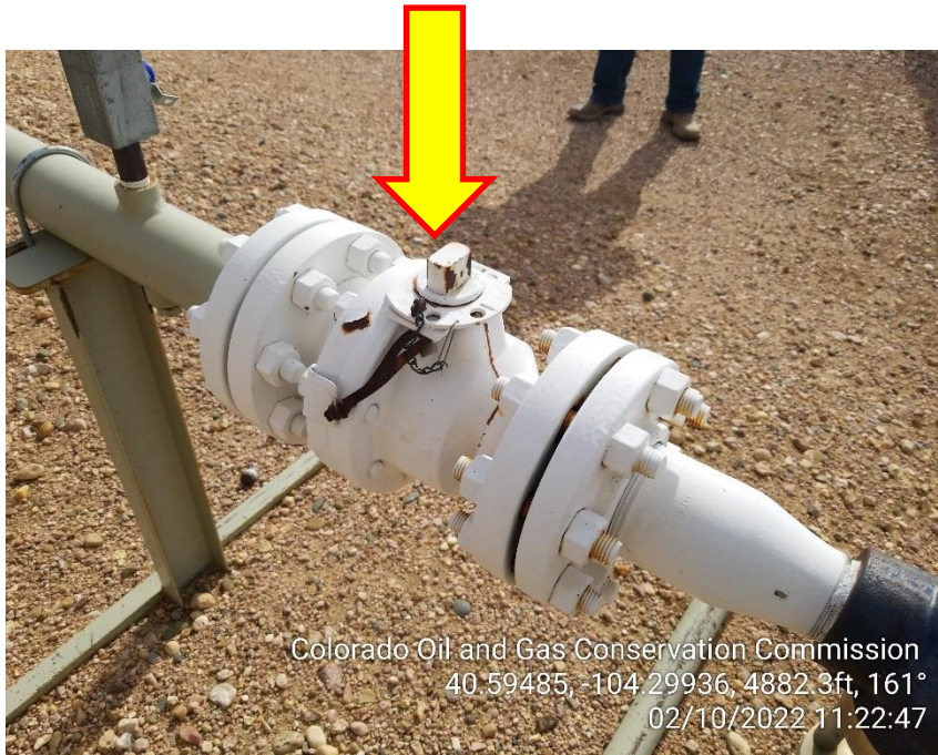
Photo 3 – Gas Line Valve Shut
