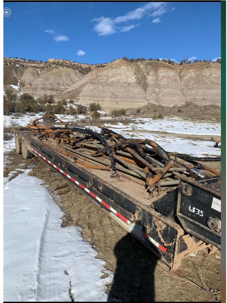
Flowlines were abandoned, dug up and removed from location
