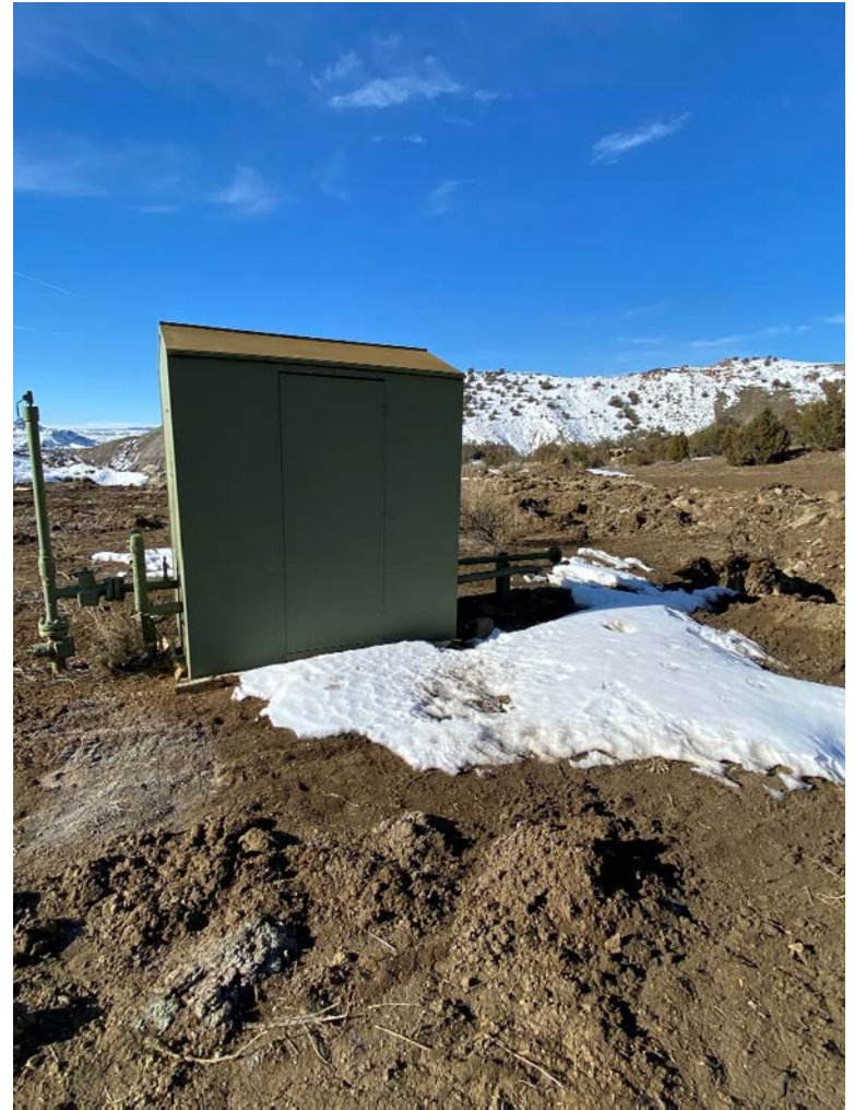
Gas meter, Building and riser will need to be removed before final reclamation can be passed
