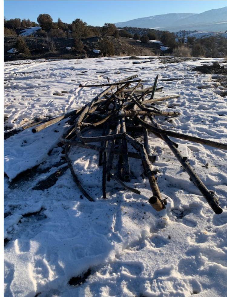
On-locations 2" flowlines dug up and removed
