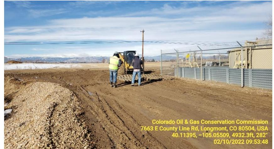
**Photo 5 Tracking pad being reset after cleaning.**
