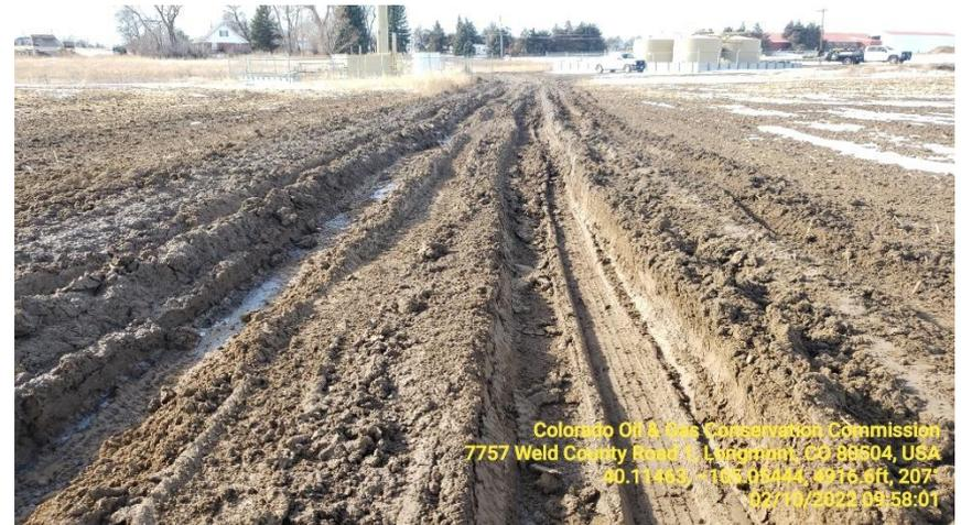
**Photo 9 Access Rd. muddy with deep ruts entering location.**
