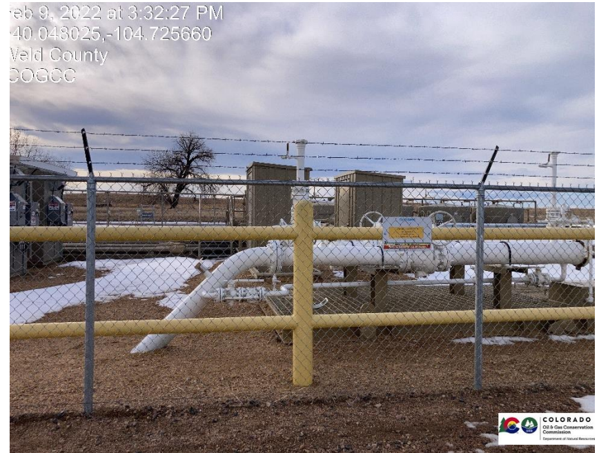
Pic 4 gas meter run
