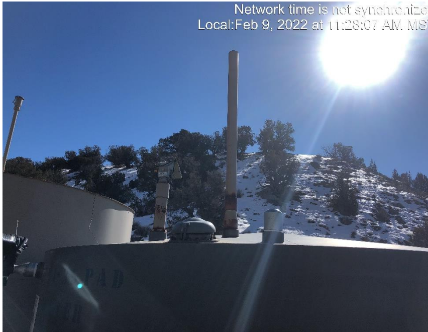
Photo #5904 Vent pipe on tank open ended.
