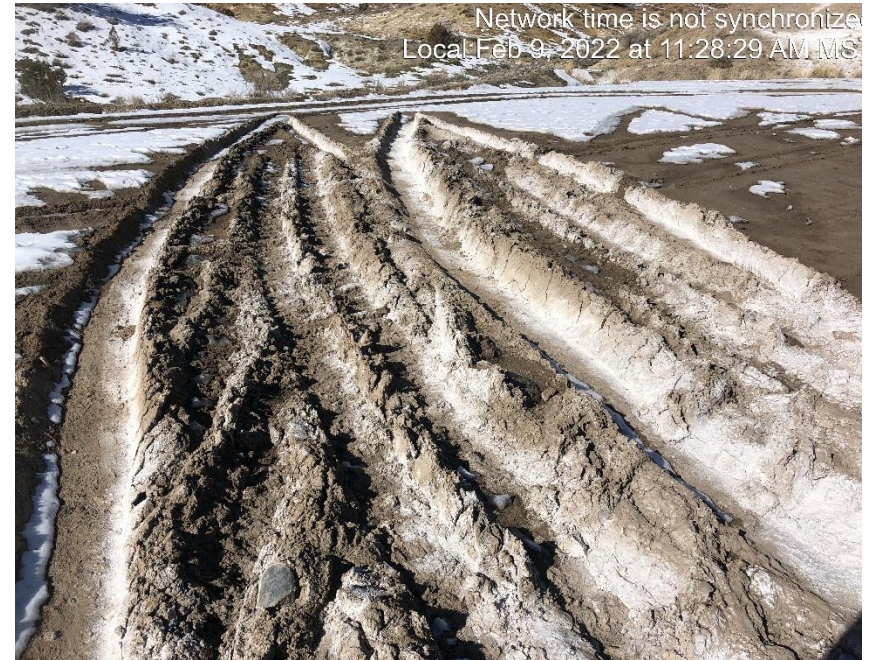
Photo #5905 Location lacks stabilization.
