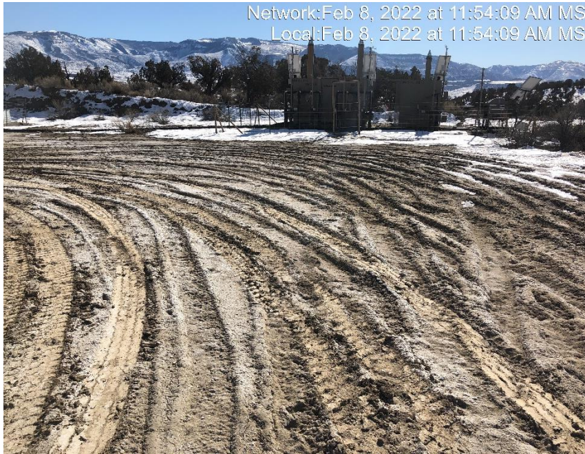
Photo #5900 Location lacks stabilization.
