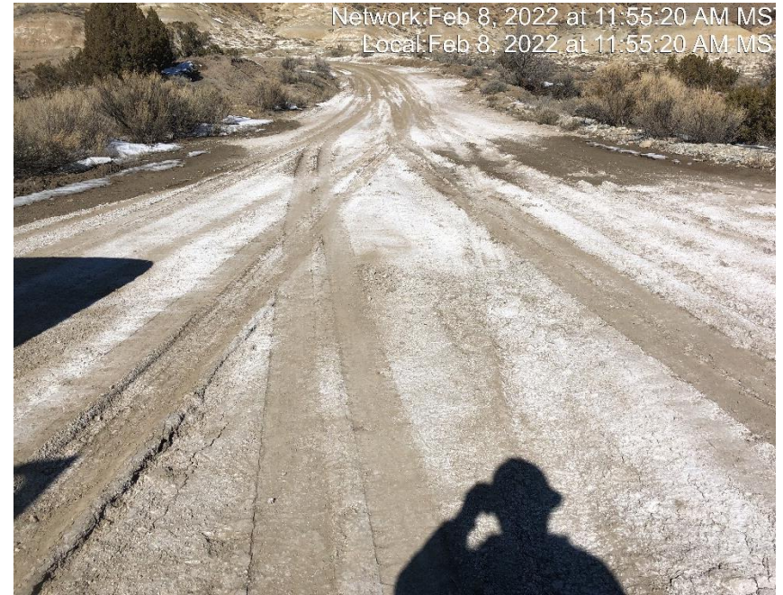
Photo #5901 Insufficient tracking BMP at entrance to location.
