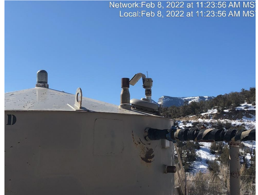
Photo #5894 Vent pipe open on tank open ended.
