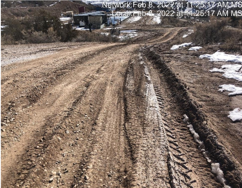
Photo #5897 Insufficient tracking BMP at entrance to location..
