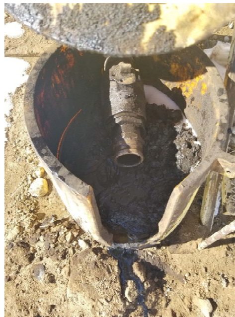
Photo 4. Drip pot overflowing.
