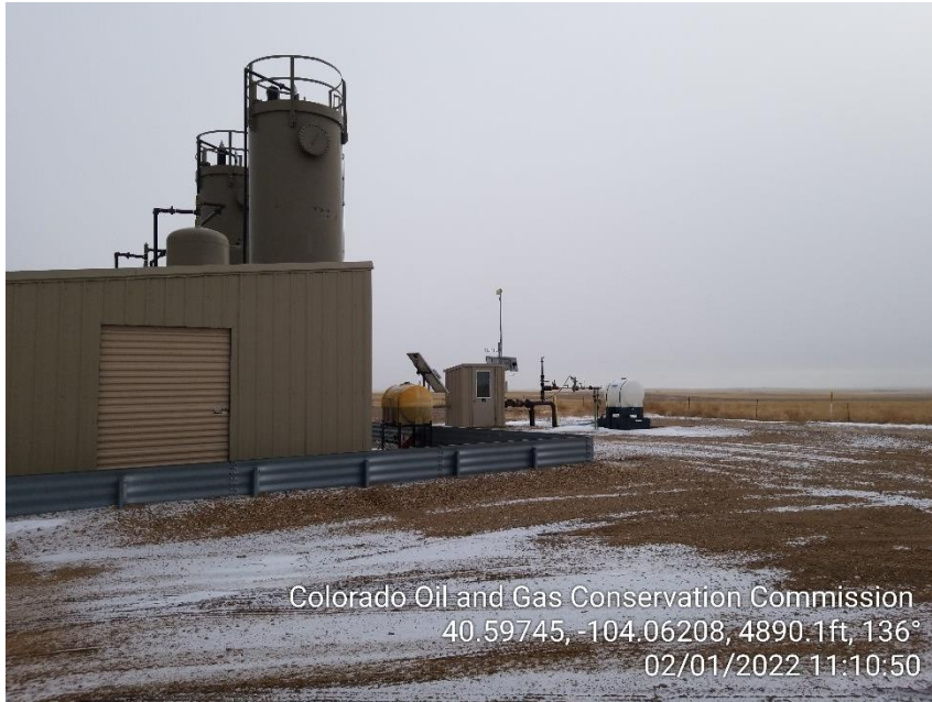
Photo 15 – Heater Treaters and Gas Meters
