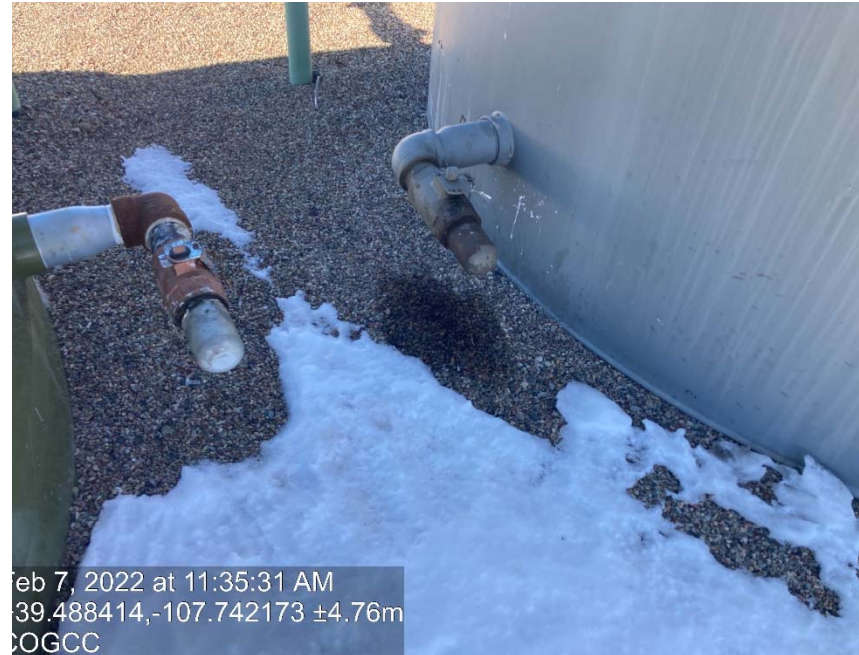
Staining under valve
