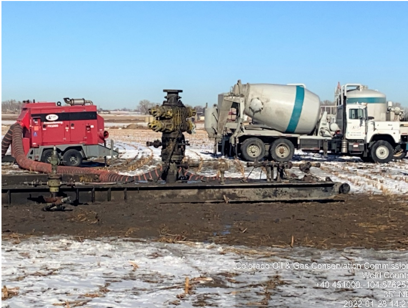
Photo #1 Uhrich 14-29 (05-123-21811) Wellsite Plugged & Abandoned | PA Plugging Operations: Cementing | WK Final cement to surface
