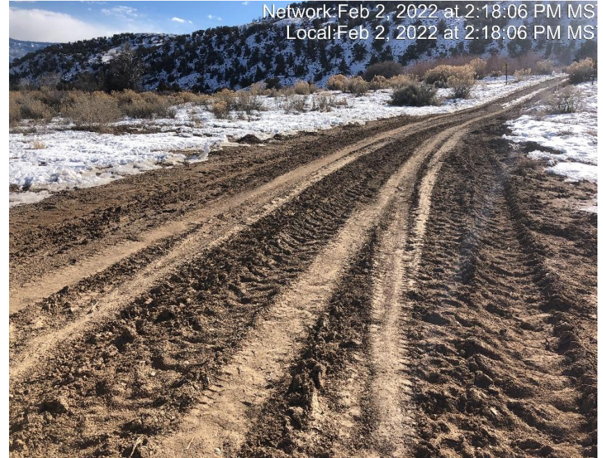
Photo #5868 Insufficient tracking BMP at entrance to location.
