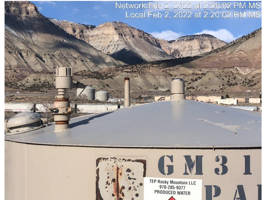
Photo #5869 Vent pipe on tank open ended.
