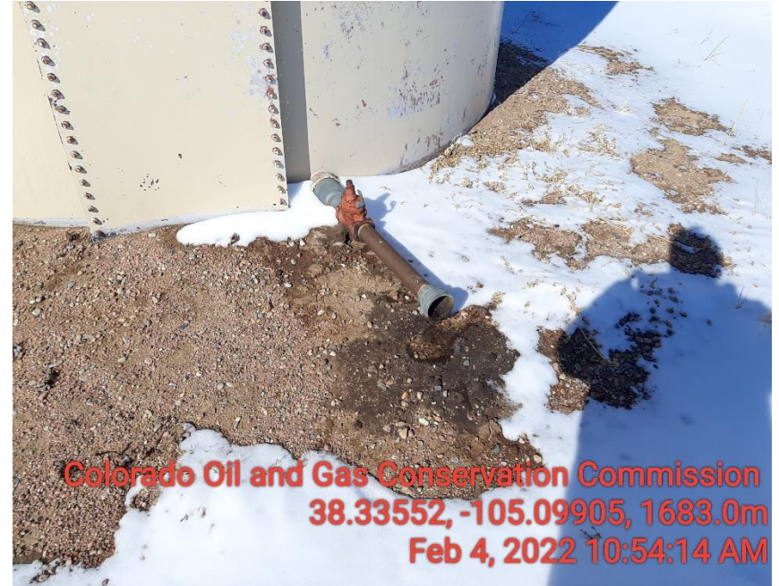
Photo 4 stained soil and mechanical issue take load out line.
