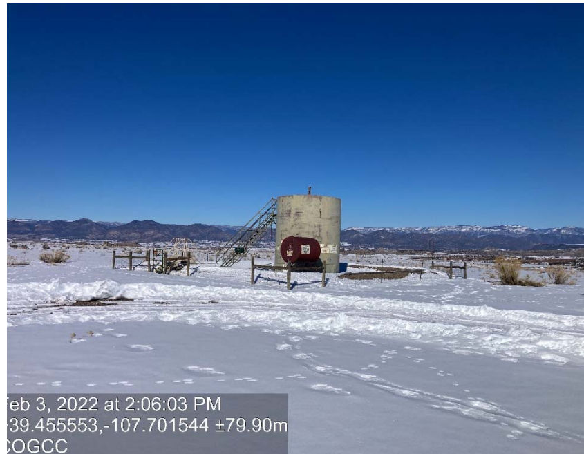
Location/lack of battery signage
