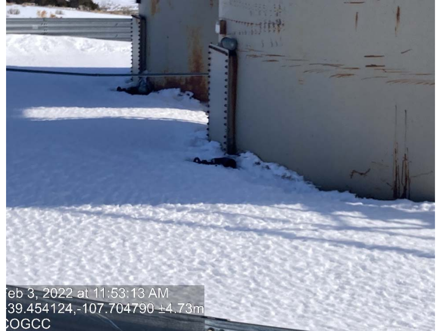
Load line missing bull plug
