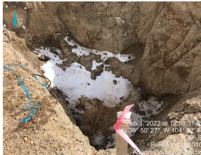
Photo#8 Open remediation work/Open hole where concrete water vault was.
