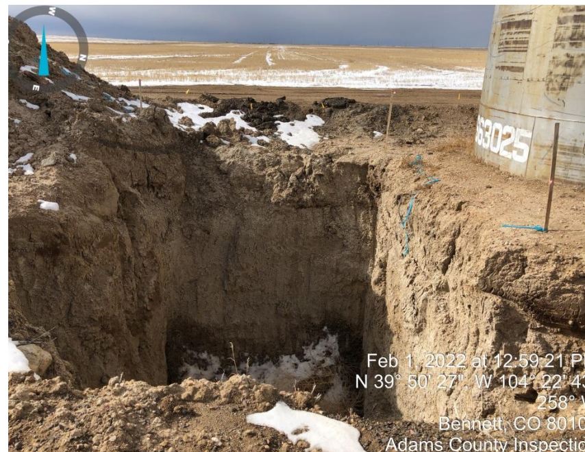
Photo#10 Open remediation work/No Safety fencing around hole.
