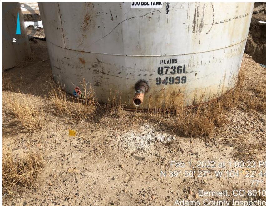
Photo#14 Corrective Action: 603.i. All loadlines will be bullplugged or capped.
