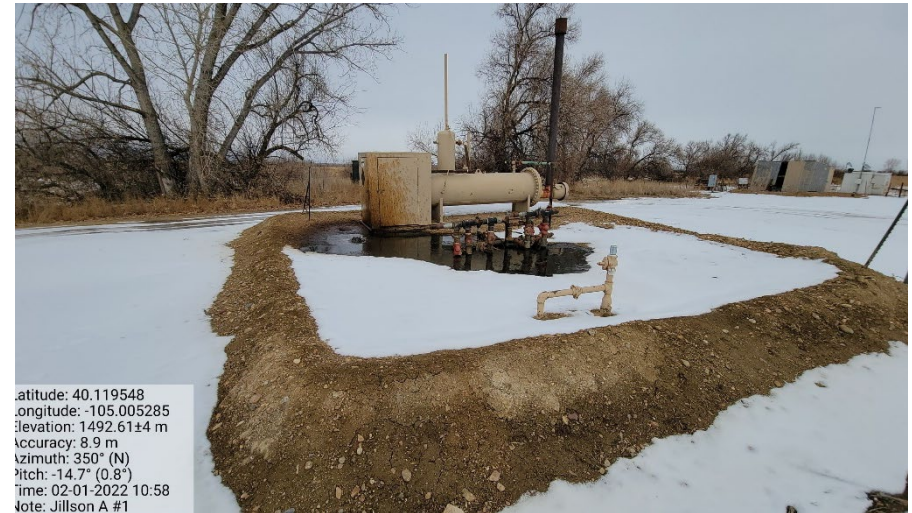
Photo 2 – Active spill at separator.
