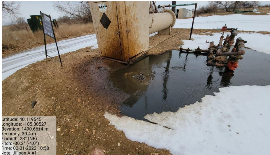
Photo 1 – Active spill at separator at Jillson A 1 Battery.
