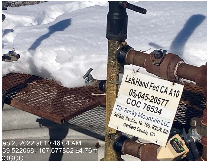
Leaking well head
