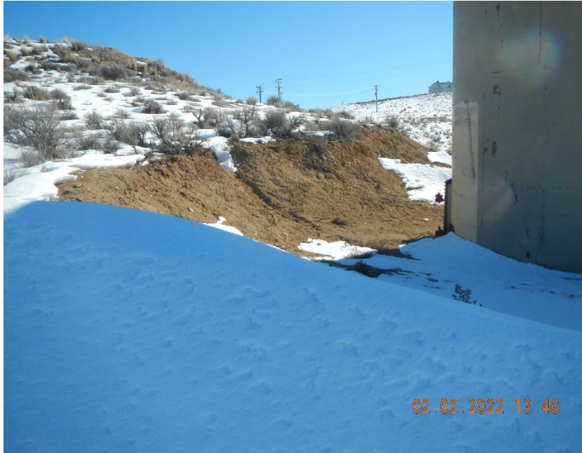
Erosion rill running into tank berm from cutslope.
