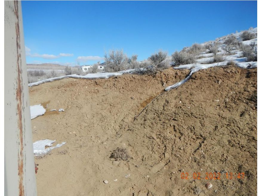
Erosion rill running into tank berm from cutslope.
