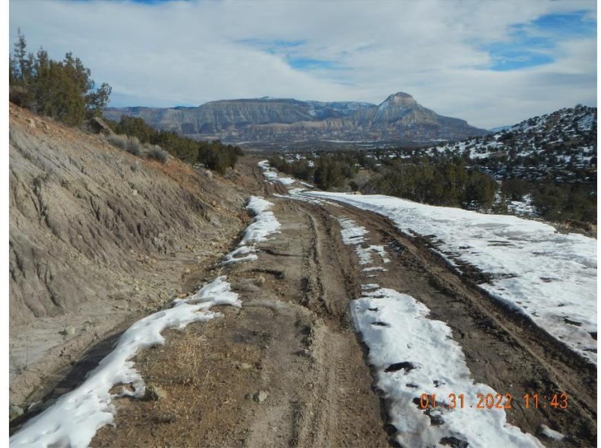
**Access road is rutted and lacks stabilization. Road ditch needs maintained.**
