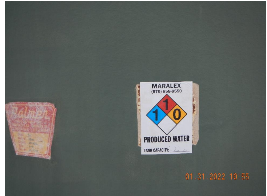
Capacity is blank on tank label.
