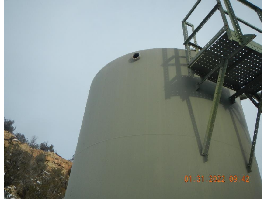
Open access hole at top of tank.
