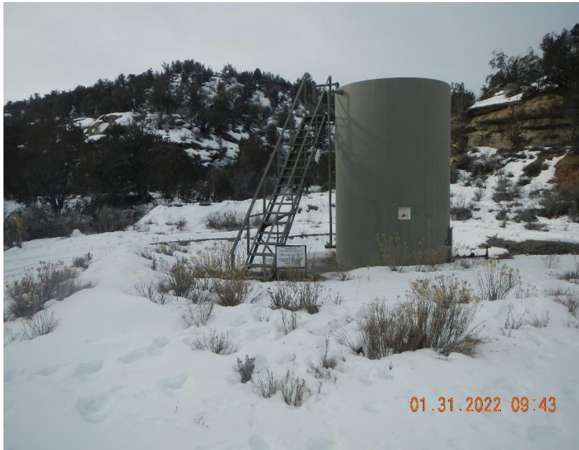
Secondary containment not adequate weeds and debris inside tank containment.
