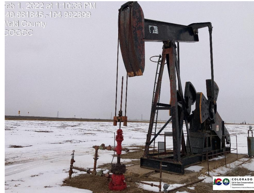
Pic 1 Wellhead, pump jack
