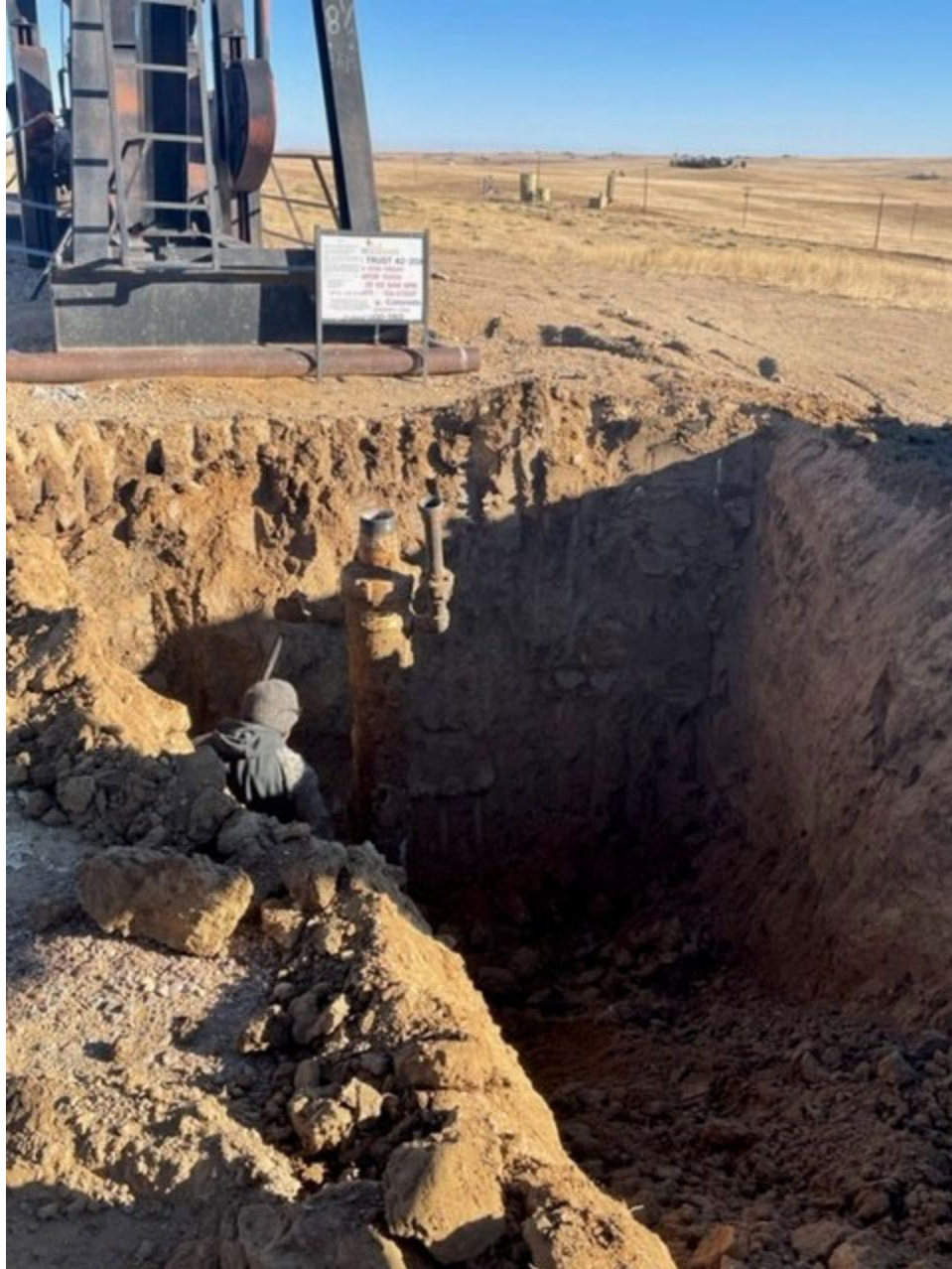
2 – Nordman Trust 42-20X – wellhead cut and cap in process
