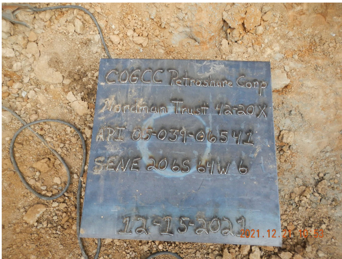
6 – Nordman Trust 42-20X – wellhead capped with nameplate
