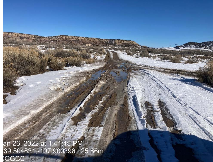
Lack of stabilization/compaction/degradation
