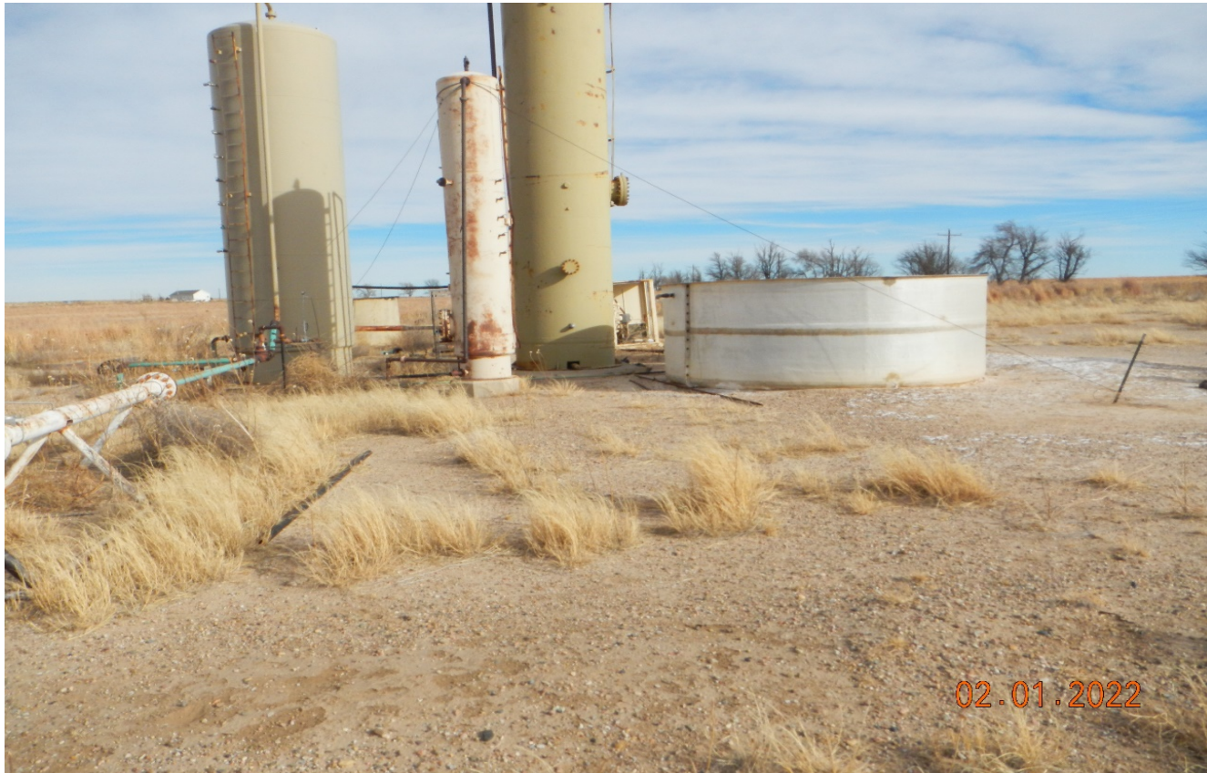
Photo 12. Facing east toward the facility.
