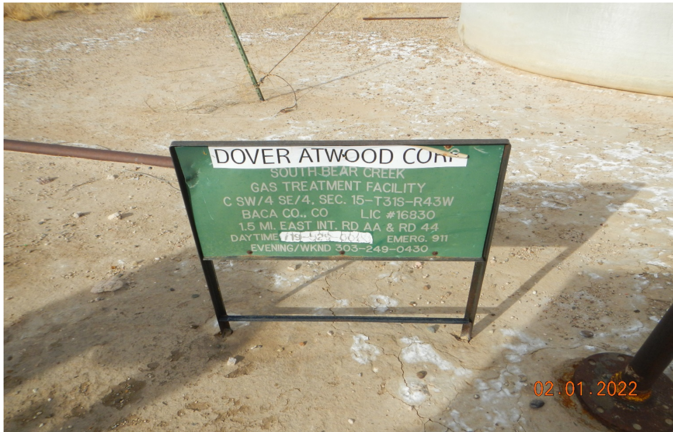
Photo 3. The facility sign is obscured behind the compressor. The emergency contact number is not valid.
