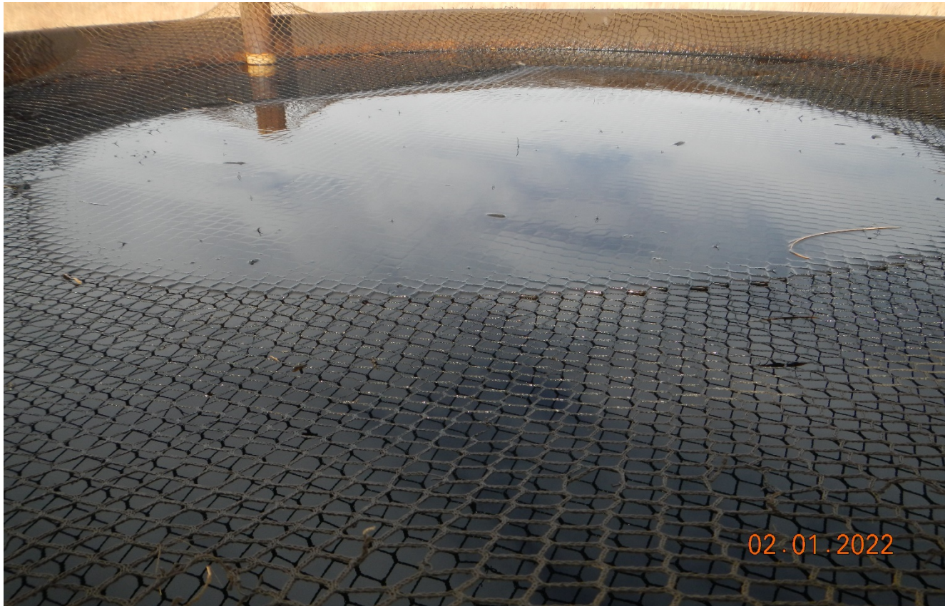
Photo 8. The liquid in the tank is near the top which could spill over. The netting is not adequate to prevent wildlife entry.
