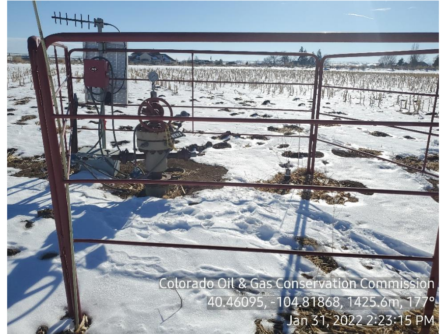
Photo 2: TA Wellhead
