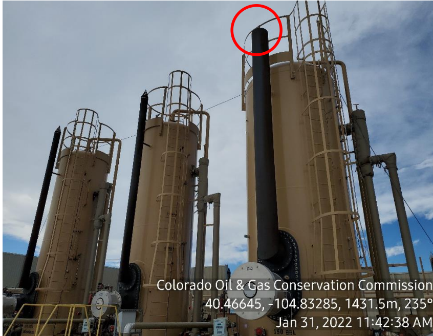
Photo 9: Missing bird protector
