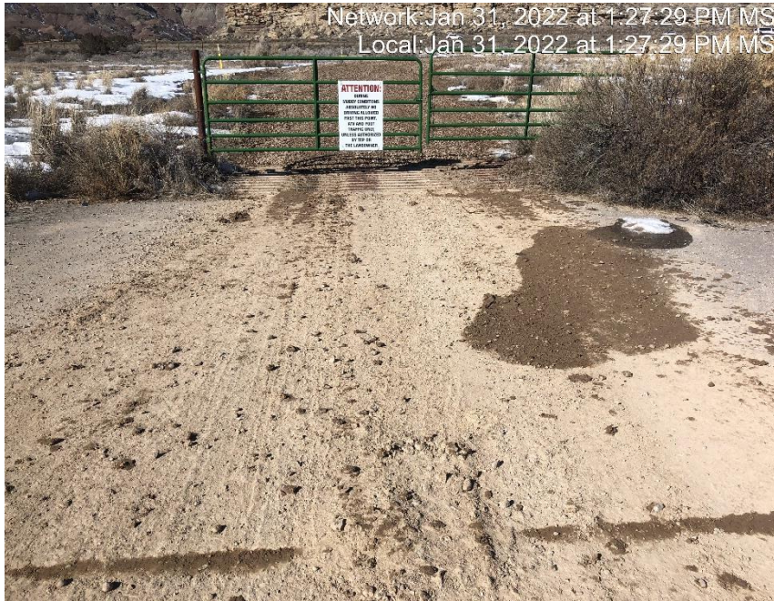
Photo #5842 Insufficient tracking BMP located at entrance to location.
