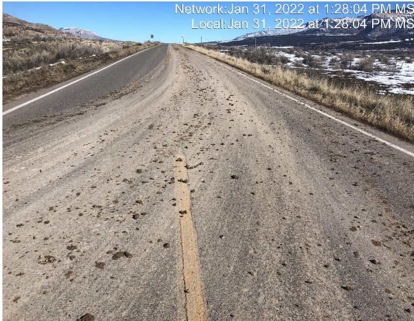
Photo #5845 Tracking occurring from location and access road for approximately 100 yards.
