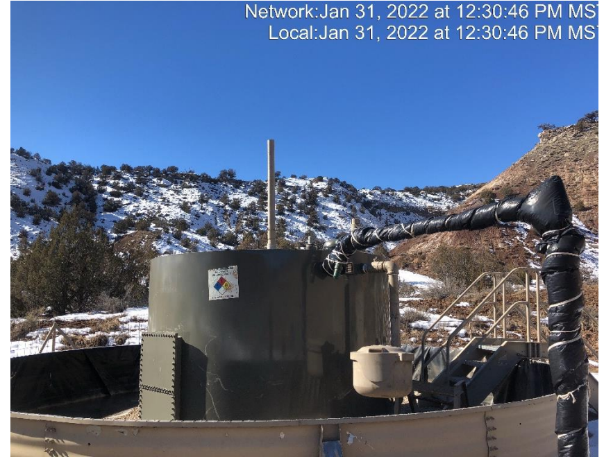
Photo #5832 Vent pipe on tank open ended.
