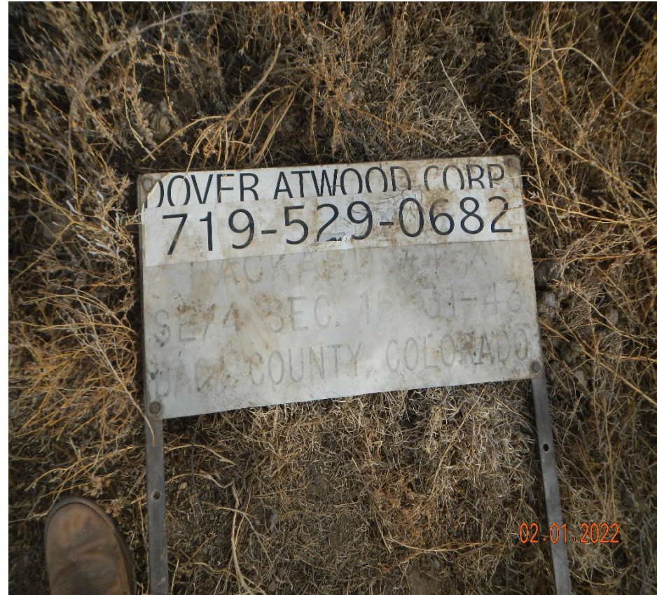
Photo 6. The emergency contact number was not valid and does not meet the signage requirements.
