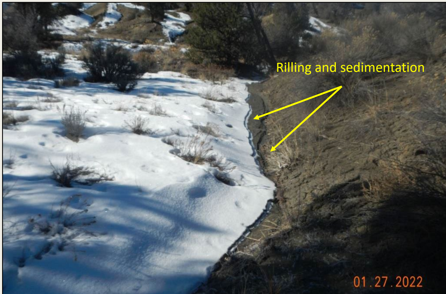
Photo 3. View of southern diversion, facing downslope, although partially snow covered, erosional rilling and sedimentation continues here.
