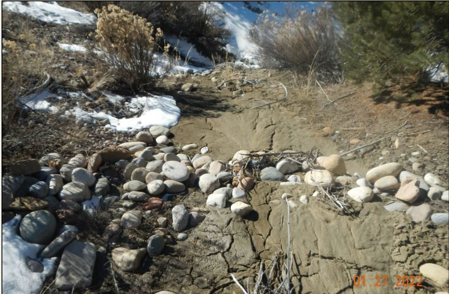
Photo 5. View of cobble BMP where stormwater flows from the access road discharge down-slope into a drainage. Diversion is full of sediment and BMP is not adequate.
