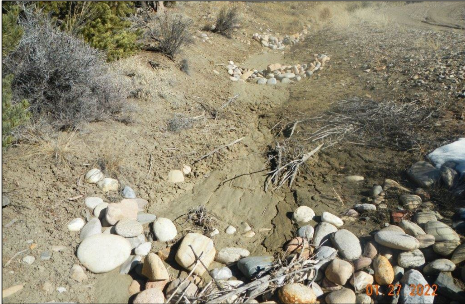
Photo 4. View of cobble BMPs along the access road, are full of sediment, are not adequately sized or properly installed.
