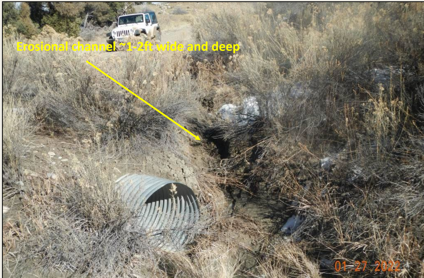
Photo 6. View of culvert inlet along the access road. Erosional down-cutting and sedimentation occurring from diverted roadside flows. Note that stream elevation is at or near inlet depth.
