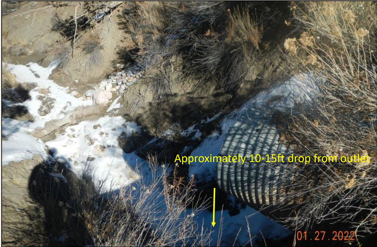
Photo 7. View of culvert outlet from culver shown in Photo 6. Outlet depth is approx 10-15ft below grade, indicating unstablized outlet and erosional down-cutting.
