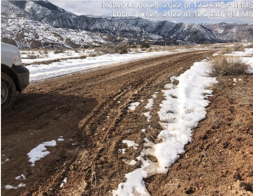
Photo #5777 Insufficient tracking BMP at entrance to location.
