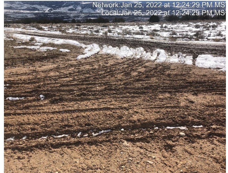
Photo #5776 Access road lacks stabilization.
