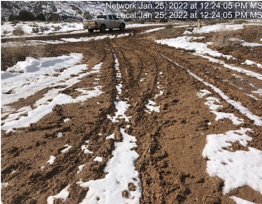
Photo #5775 Access road lacks stabilization.
