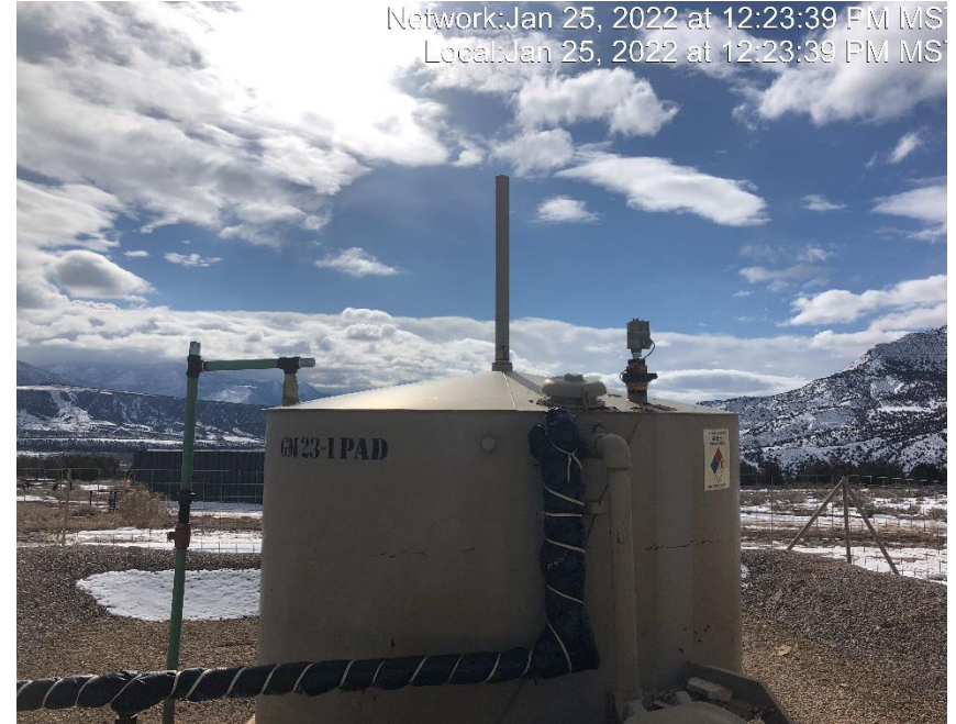
Photo #5774 Vent pipe on tank open ended.
