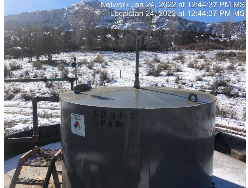
Photo #5766 Vent pipe on tank open ended.
