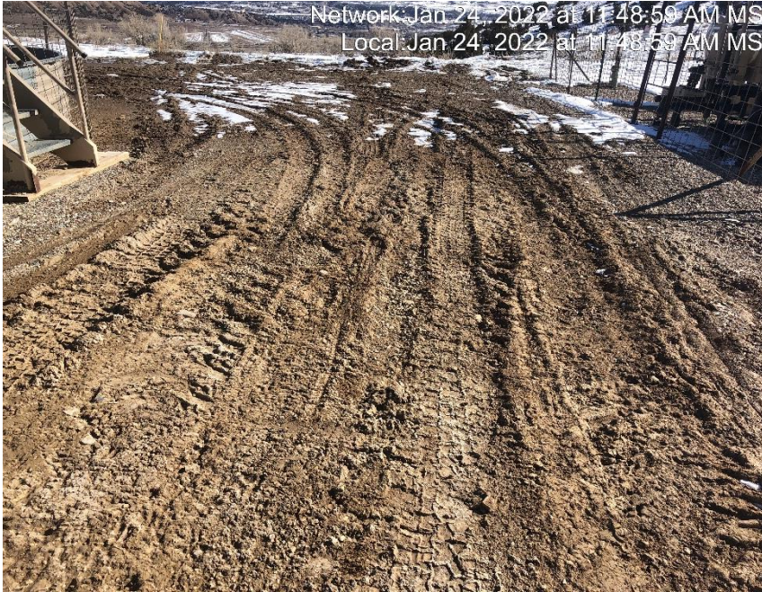
Photo #5762 Location lacks stabilization.
