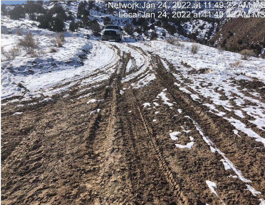
Photo #5764 Insufficient tacking BMP at entrance to location.
