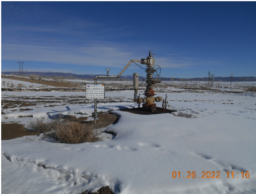
Injection wellhead
