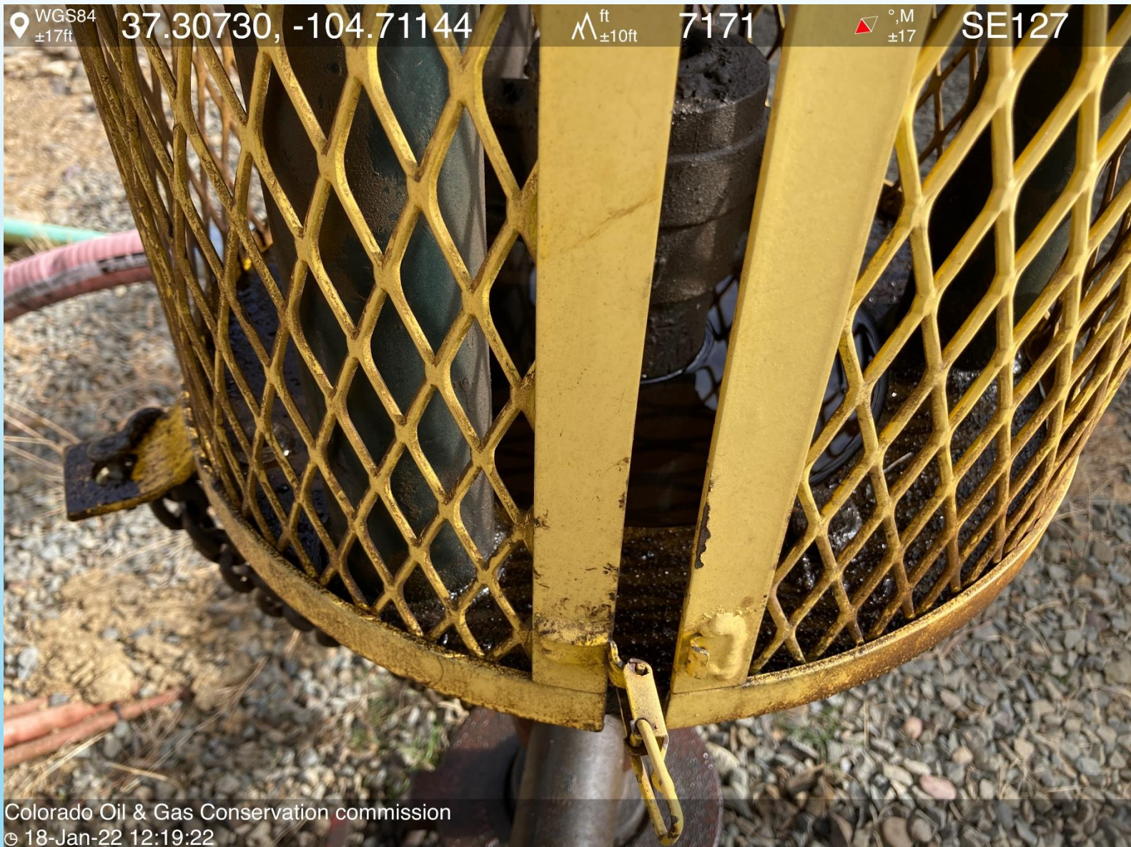
PHOTO 4: THERE IS WHAT APPEARS TO BE OIL POOLING ON BOTTOM DRIVEHEAD PLATE.
